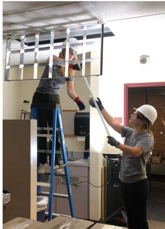
ASCP Staff installing LED lights.
