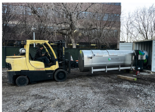
Installation of Bio Speed M4 In-Vessel Unit.
