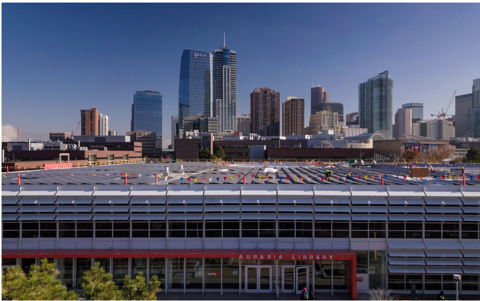
The completed solar array under the Denver skyline
