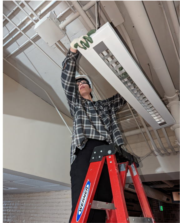
Piper Malczewski swaps out a mercury light rod for an LED light rod
